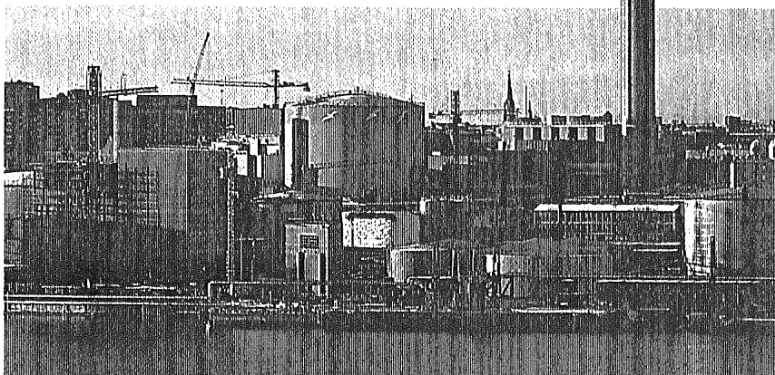
The pressurised fluidised bed (PFBC) coal fired combined cycle plant at Värtan, near Stockholm City, is equipped with a GBA generator. The generator is also used as a frequency controlled synchronous motor for starting of the plant.
